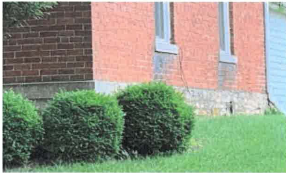
Example of original stone foundation
