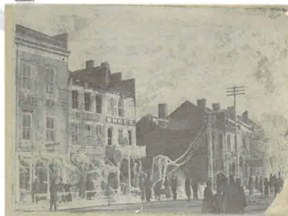
Commercial Row - N. Market Street (March 1900)
